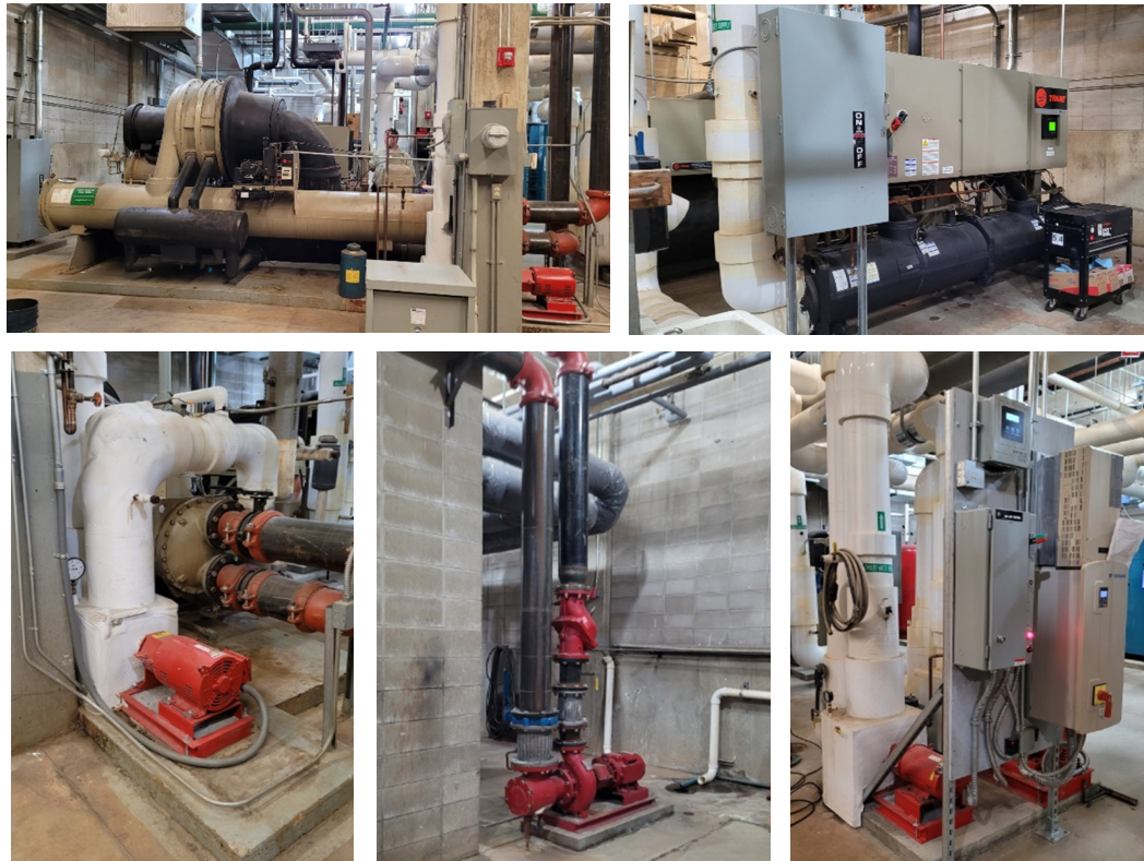
Figure 2-19 Top Left: Chiller No.1 (Water-Cooled), Top Right: Chiller No. 2 (Air-Cooled), Bottom Left: Chiller No. 1 (Primary-Pump), Bottom Middle: Water Condenser, Bottom Right: Chiller No. 2 & Building Loop Pumps
