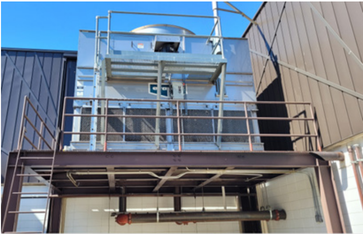
Figure 2-18 Cooling Tower
