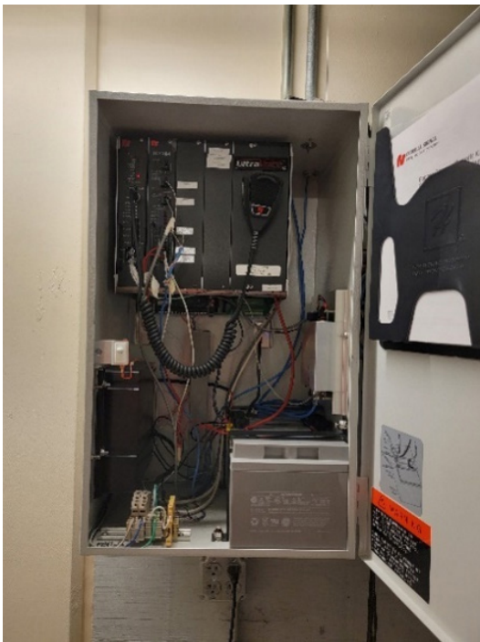
Figure 2-28 TOA System Head End
