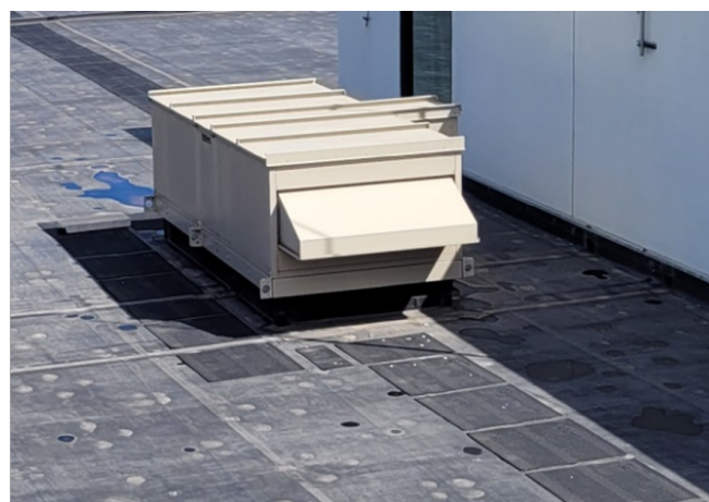
Figure 2-20 Roof-Mounted Air Handling Units
