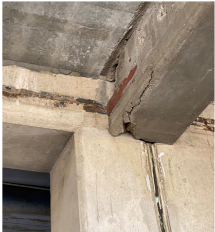
Figure 2-14 Damaged Concrete Floor Beam
