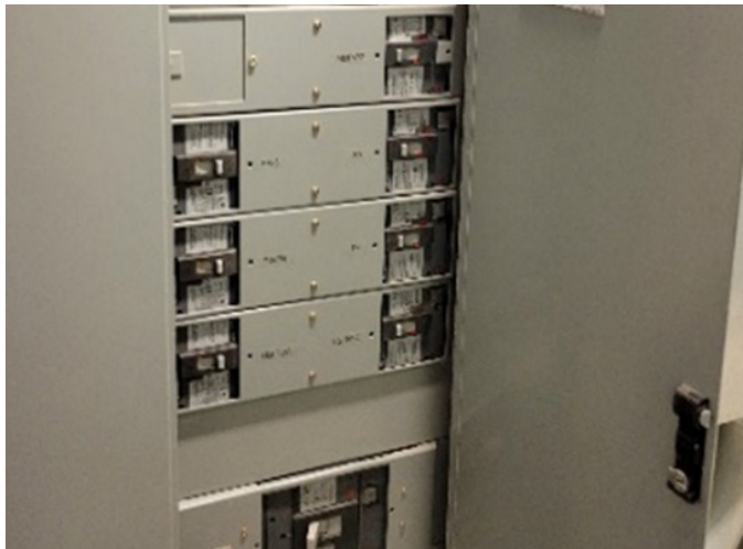
Figure 2-23 Main Service Switchboard MSB1-House/480V
