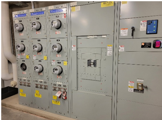
Figure 2-23 Main Service Switchboard MSB1-House/480V
