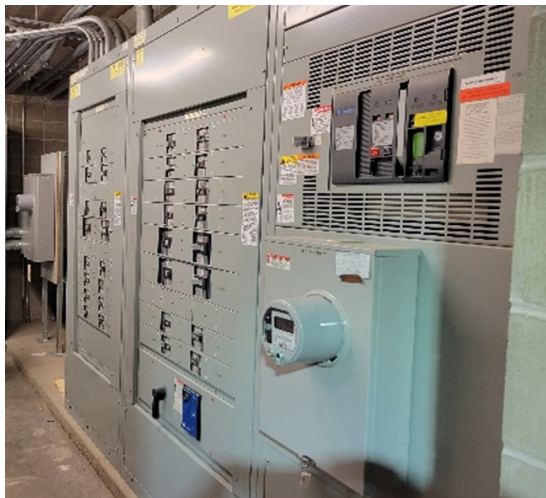
Figure 2-24 Main Service Switchboard Kitchen 480V
