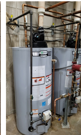
Figure 2-22 Water Heaters
