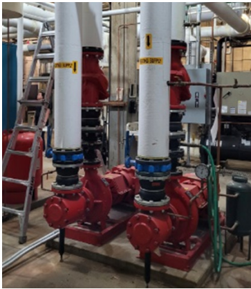
Figure 2-17 Hot Water Pumps
