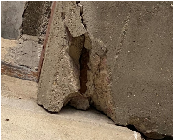
Figure 2-15 Rusting Rebar Showing Through Large Crack in Beam
