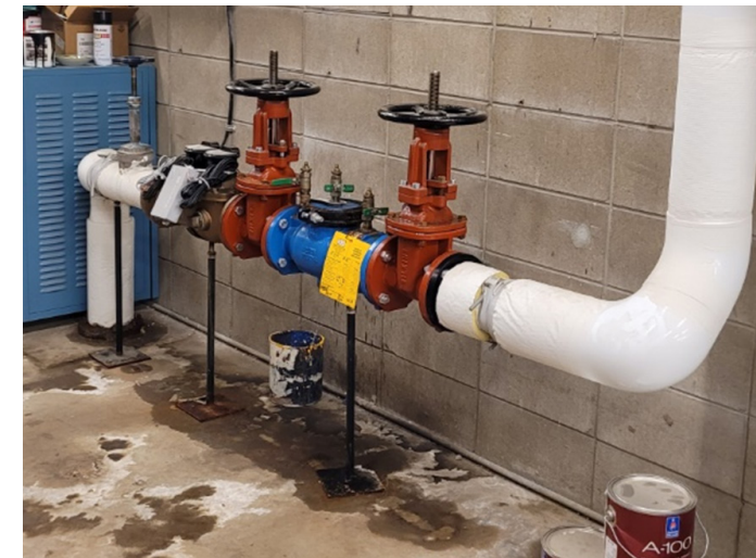
Figure 2-21 Domestic Water Service
